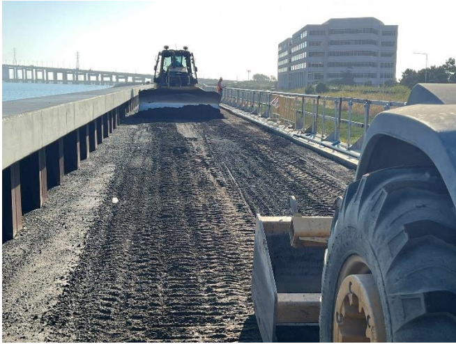
Fine grading on area North of the San Mateo Bridge
